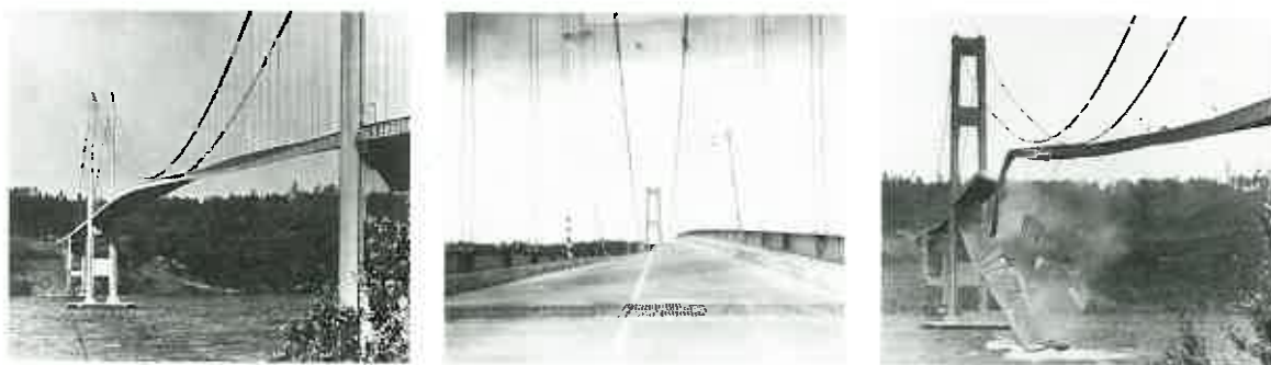
Fig. 26-12 In 1940, four months after being completed, the Tacoma Narrows Bridge in the state of Washington was destroyed by wind-generated resonance. The mild gale produced a fluctuating force in resonance with the natural frequency of the bridge, steadily increasing the amplitude over several hours until the bridge collapsed.
